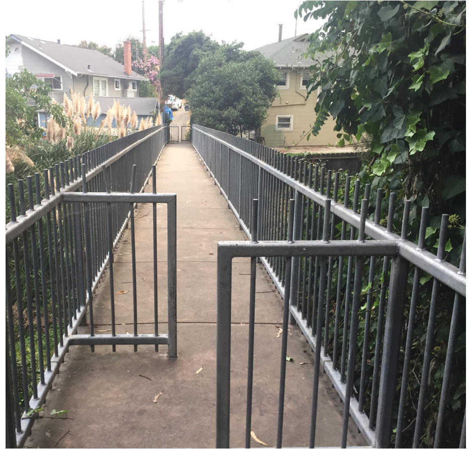
The pedestrian bridge over the San Leandro Creek.
