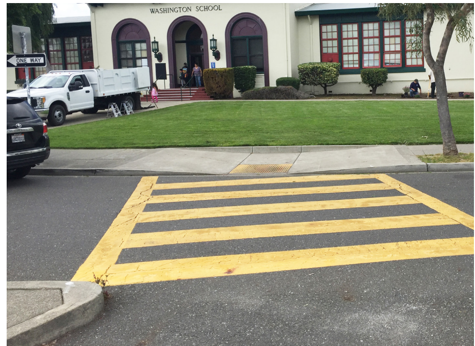
A crossing over a free right turn lane in front of Washington Elementary.
