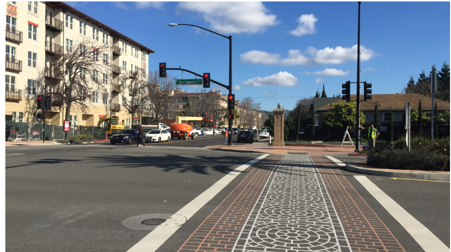
Recently improved pedestrian facilities at W Juana and San Leandro Boulevard
