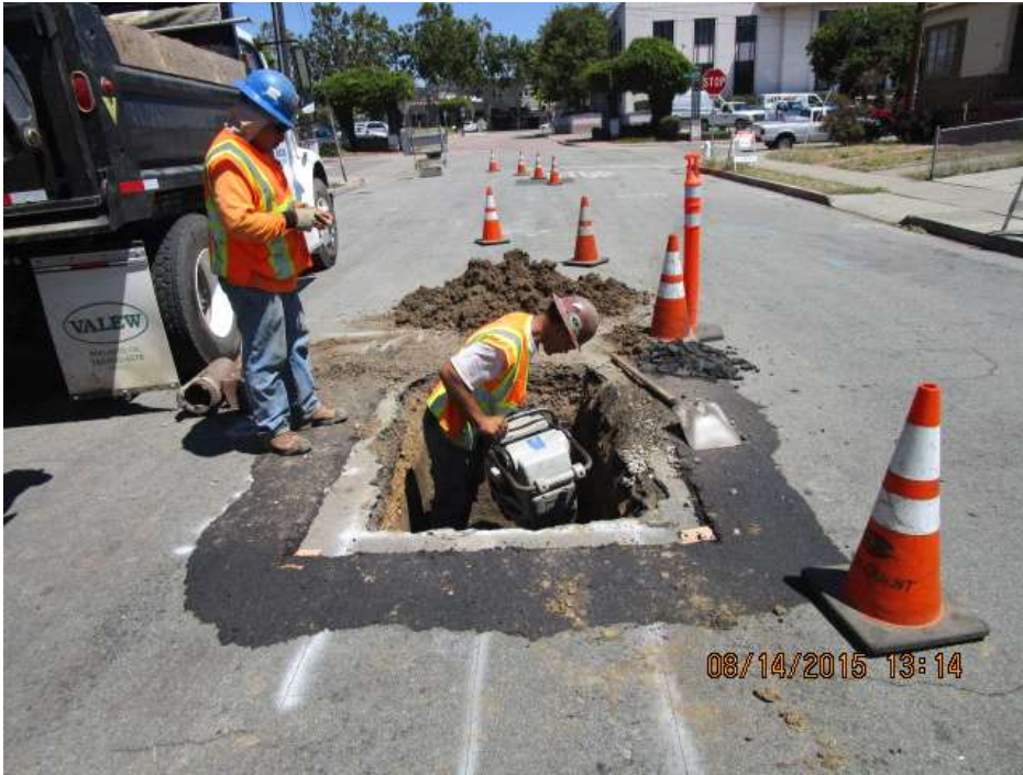
Sanitary sewer pipe repair on Lorraine Blvd.
