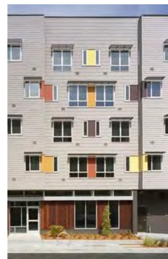
3. Cement Plank Siding
