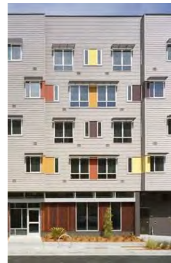
3. Cement Plank Siding
