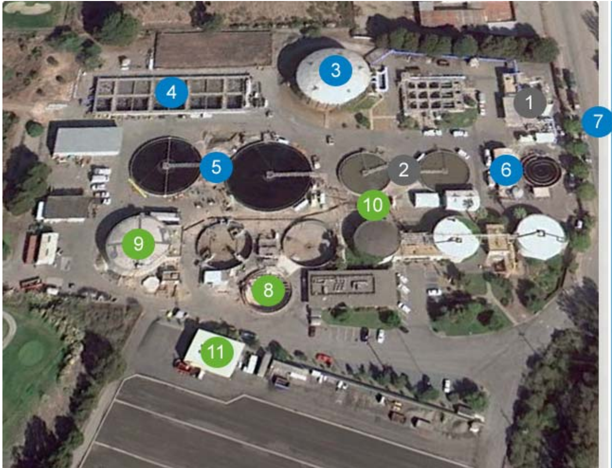
Figure 1.2.1 -- Aerial View of the San Leandro WWTF
