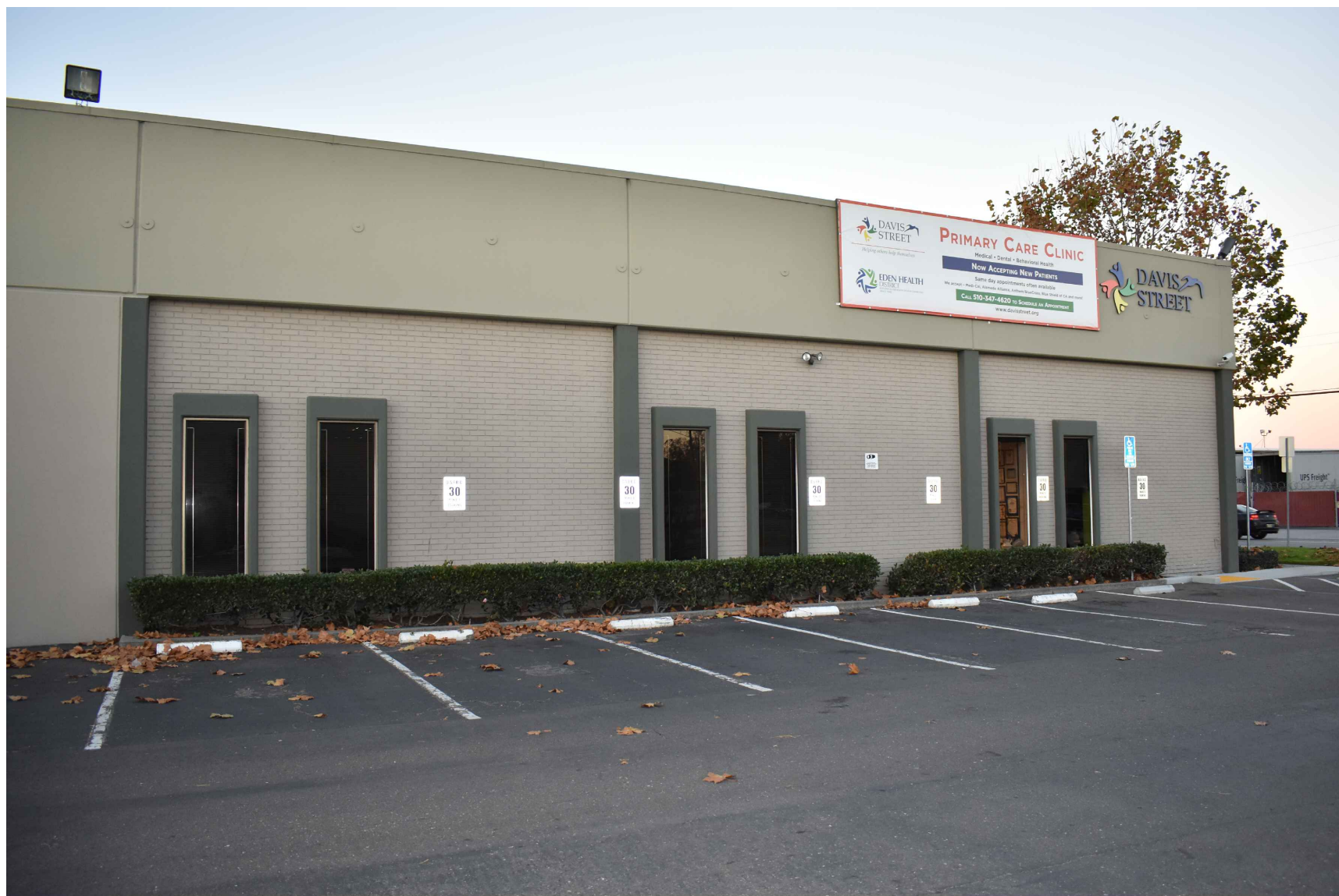
EXISTING PHOTO LOOKING NORTH-WEST
