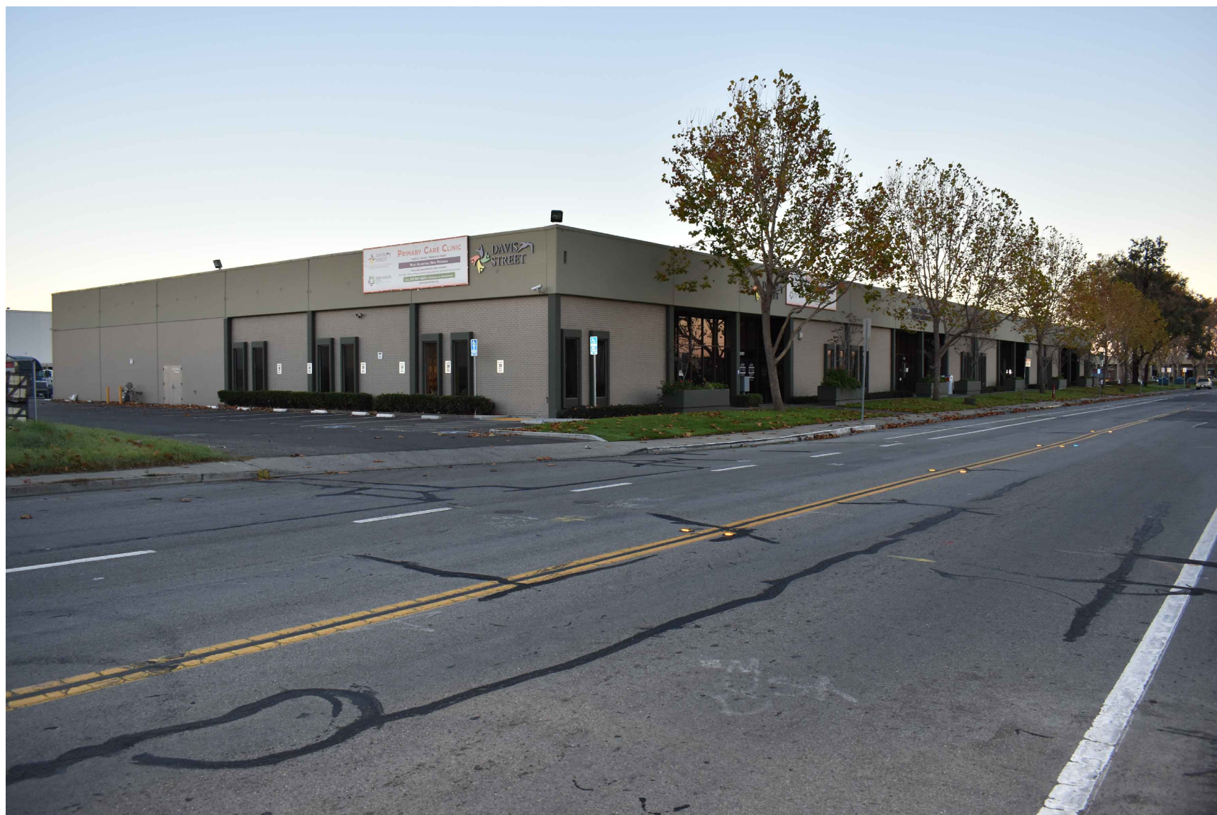
EXISTING PHOTO LOOKING SOUTH-WEST
