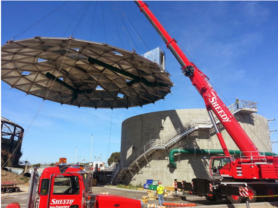
Construction of sewage treatment facilities
