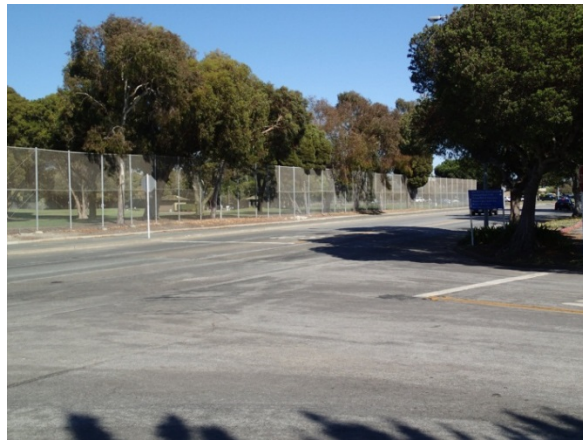
Unmarked crosswalk on Monarch Bay Drive
