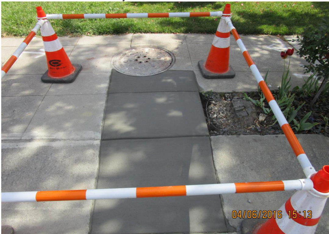
Sidewalk restoration on Farrelly Drive
