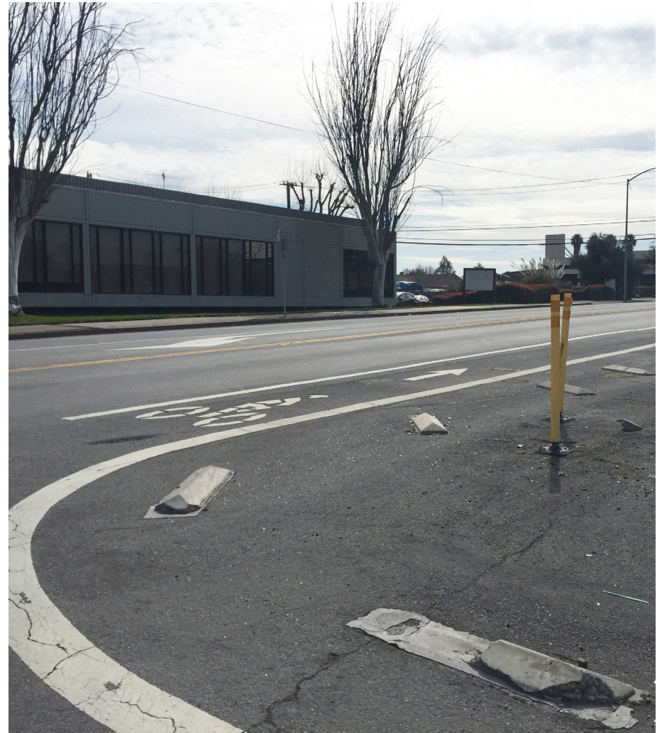
A segment of bike lane near the Kaiser Medical Center area.
