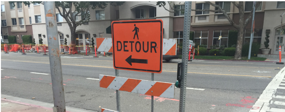
Construction along East 14th Street for East Bay BRT.
