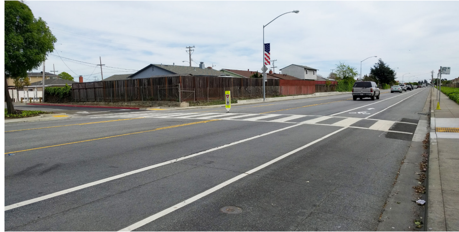
Wicks Boulevard: Existing Class II facilities are recommended to be updated to Class IV facilities.
