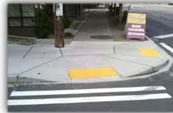
Accessible curb ramps
