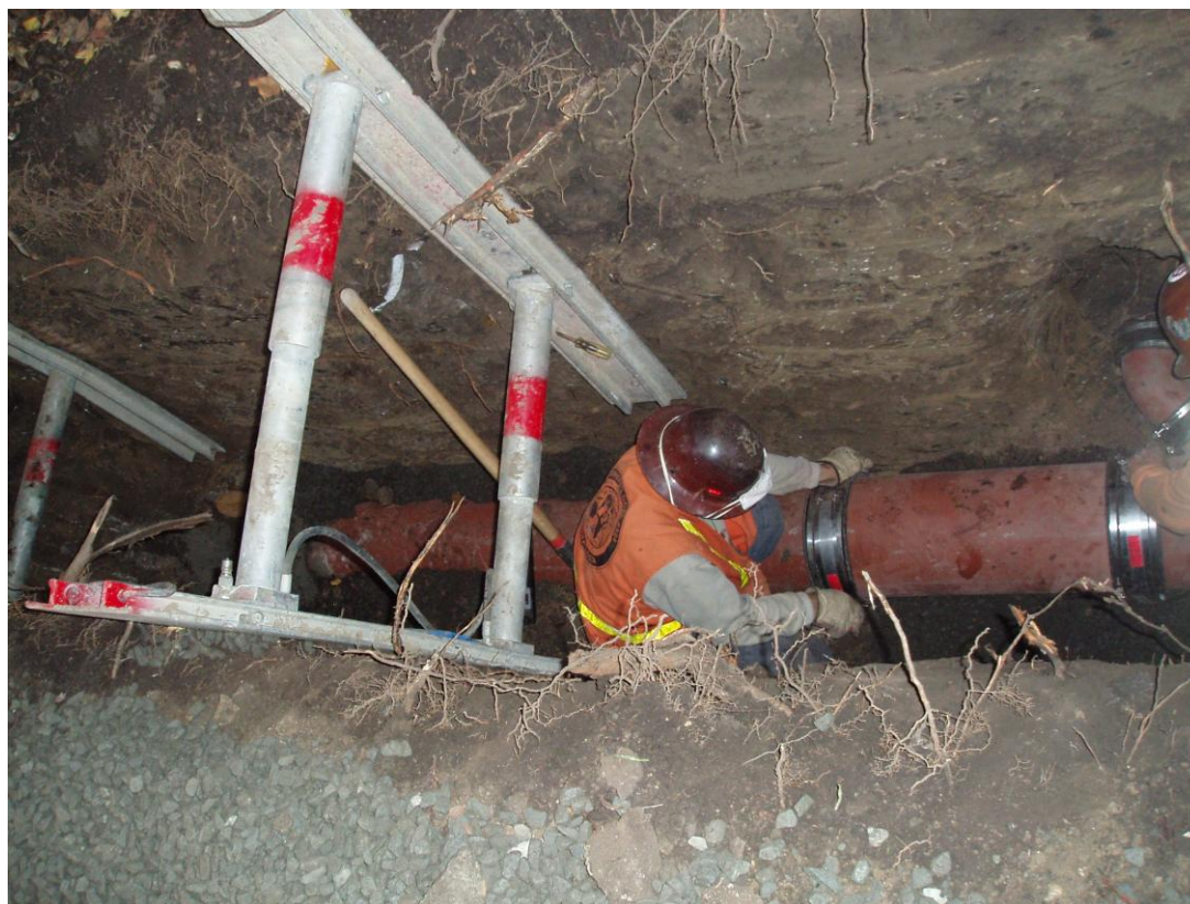
Sanitary Pipe Replacement
