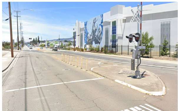
Railroad crossing locations often have gaps in pedestrian and bicycle facilities.
