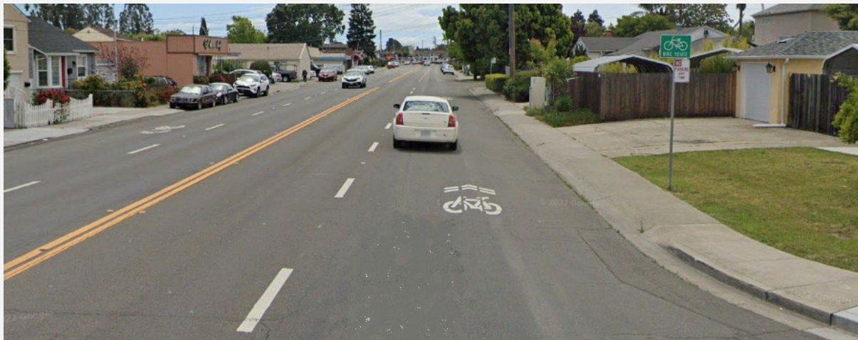
From top to bottom: (1) A bicycle boulevard on Virginia Street in Berkeley. (2) A bicycle route on 150th Avenue in San Leandro.
