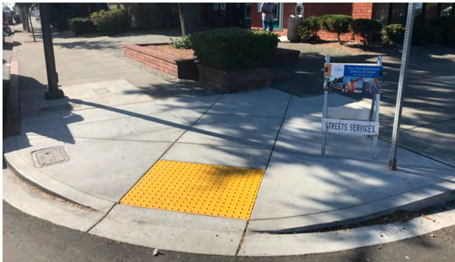
Curb Ramp Construction
