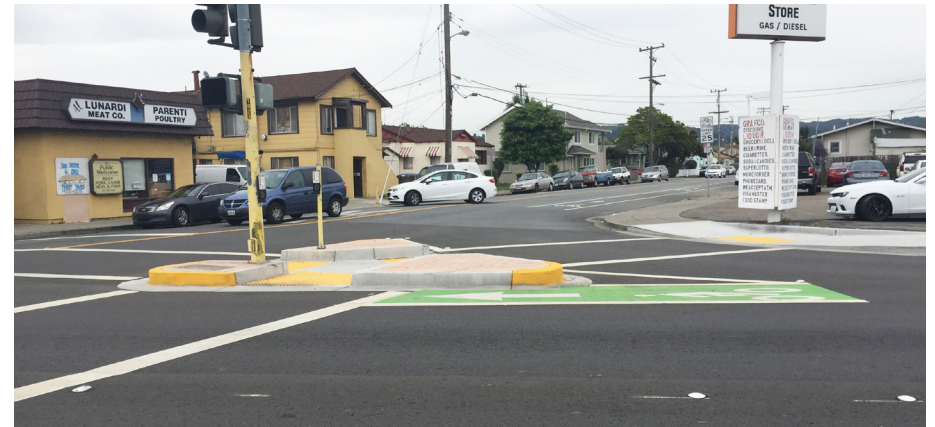
A pork chop island with free right turn lane and green bike lane at the intersection of San Leandro Boulevard and Williams Street.
