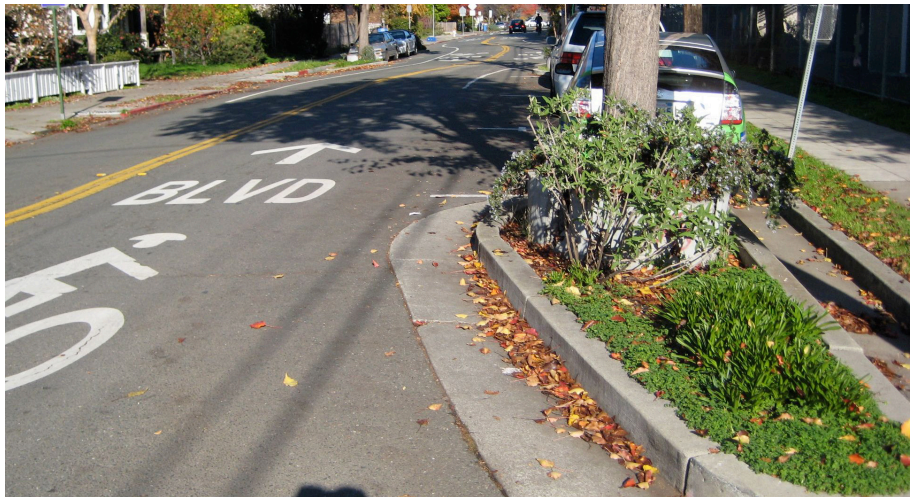
A bicycle boulevard in Berkeley that has been designed with pavement markings and a striped chicane.
