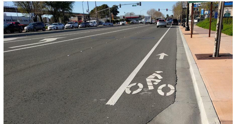
A segment of bike lane along San Leandro Boulevard.
