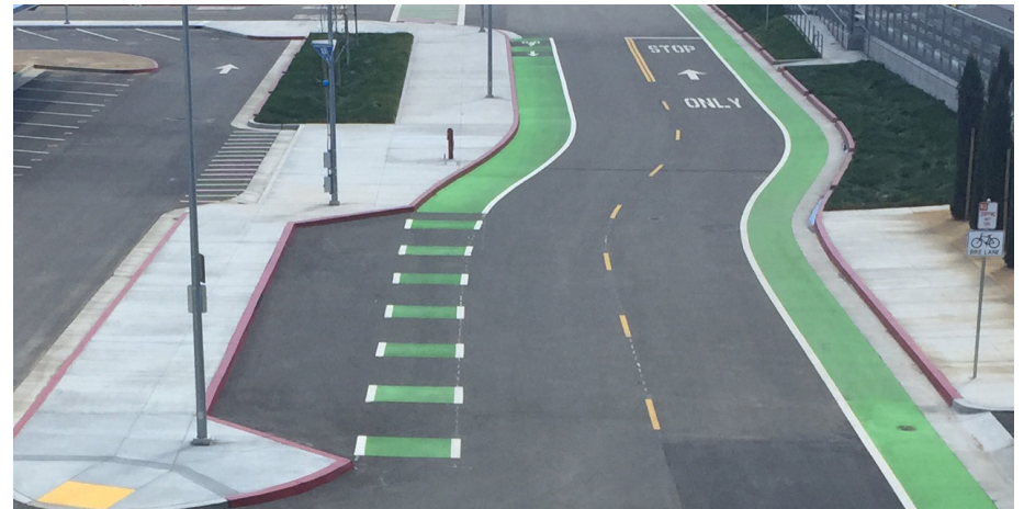
Conflict markings indicate areas where traffic mixes with bike lanes.
