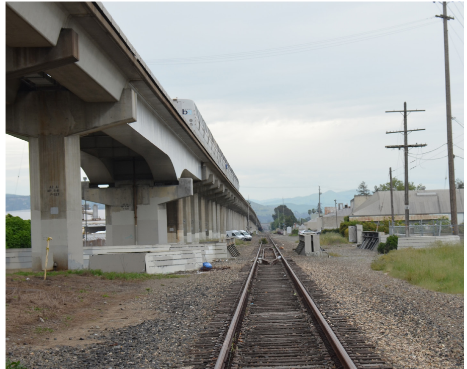
Part of the potential alignment of the East Bay Greenway, which would be a Class I shared-use path.
