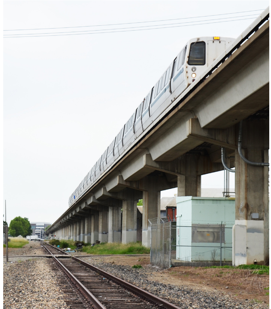
Part of the potential East Bay Greenway alignment shared with Union Pacific. Photo taken between Bay Fair and San Leandro BART Stations, near Washington Avenue.
