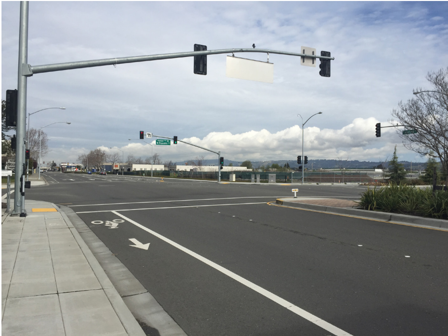
A Class II bike lane on Merced Boulevard in front of Kaiser Medical Center.
