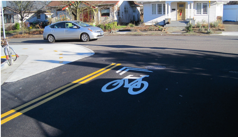
An example of sharrows with angled arrows directing riders where the bicycle route continues.
