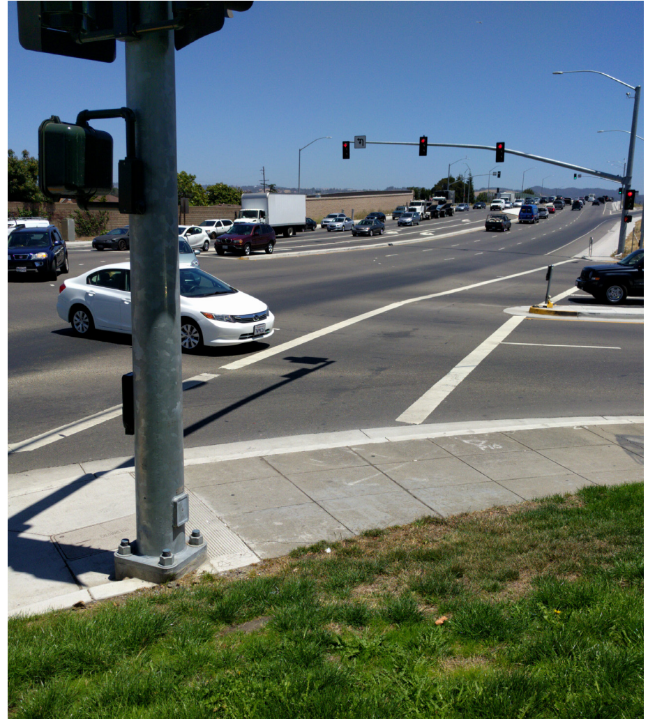
Davis Street and I-880 interchange from the Westgate Center.
