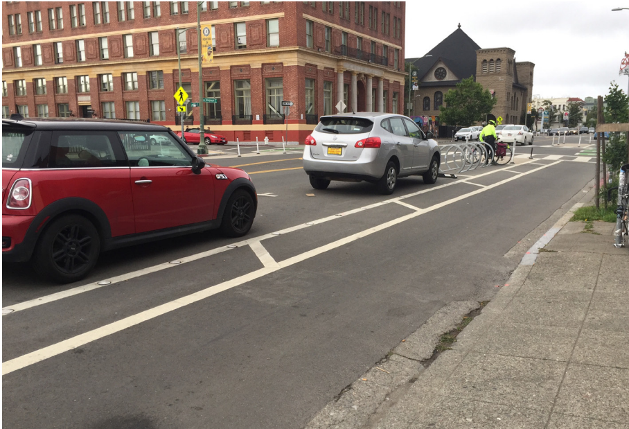
A Class IV separated bikeway in Oakland on Telegraph Avenue. This bikeway is separated using both parked cars and bicycle parking.
