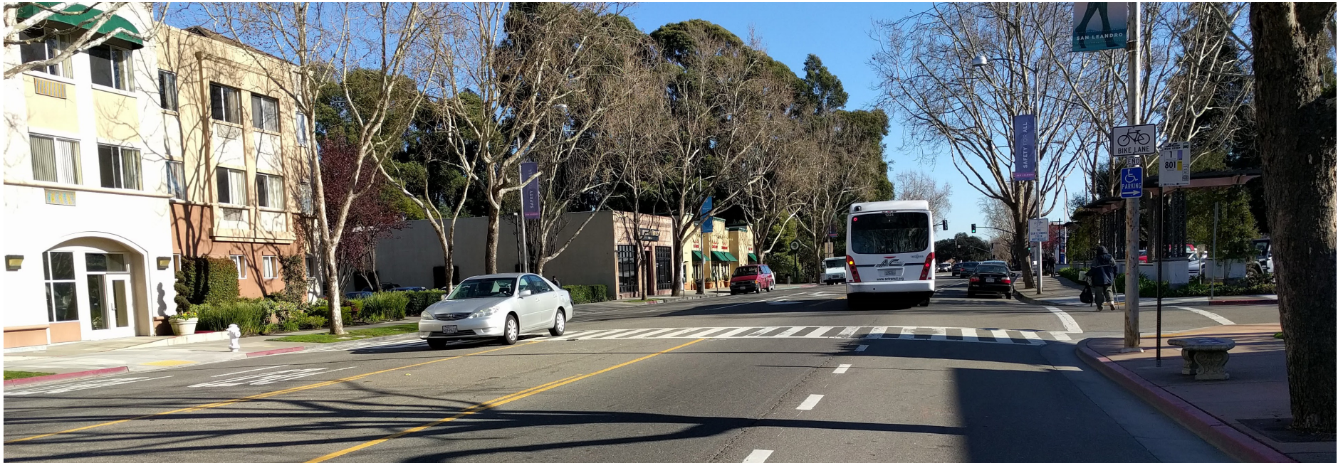
East 14th Street in front of San Leandro City Hall and the Carlton Senior Living facility. (This segment of East 14th Street was recently reconfigured as a part of the East Bay BRT project).
