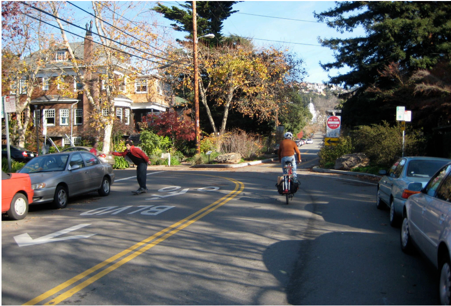
A bicycle boulevard in Berkeley with signage, roadway markings, and a partial street closure.
