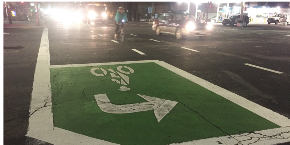
A bike box at the intersection of Grand Avenue and Telegraph Avenue in Oakland.
