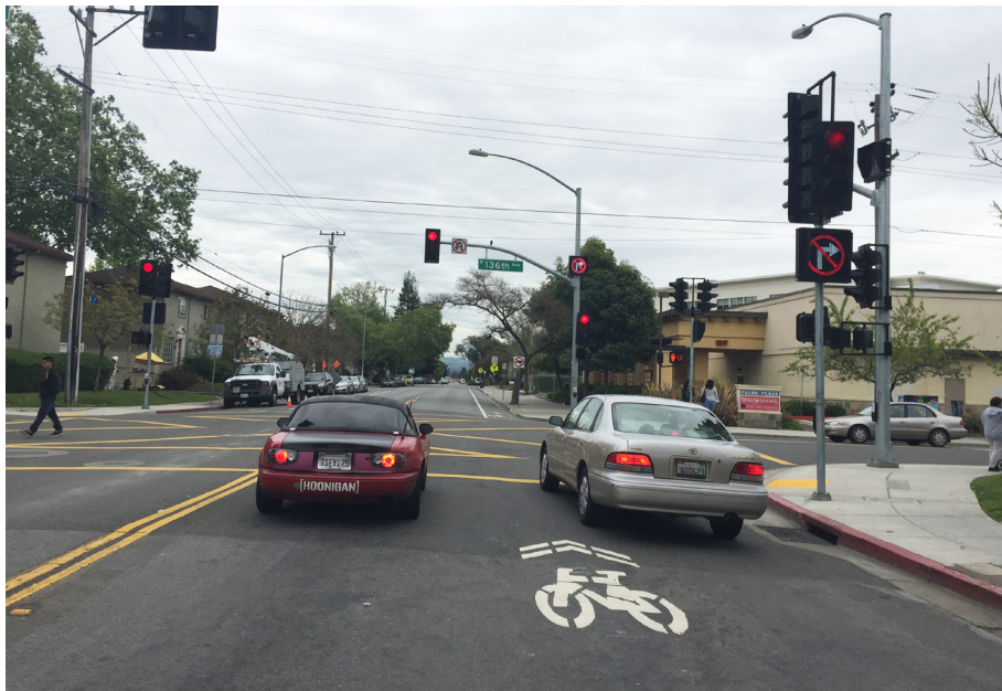
Sharrows on a segment of Bancroft Avenue near San Leandro High School.
