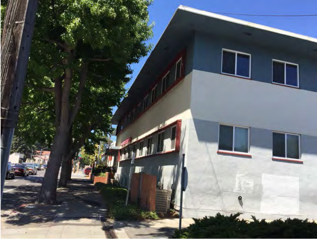
Photograph 2. View north of east and south elevations
