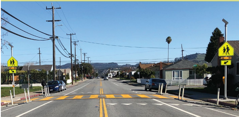
Rectangular Rapid Flashing Beacon
