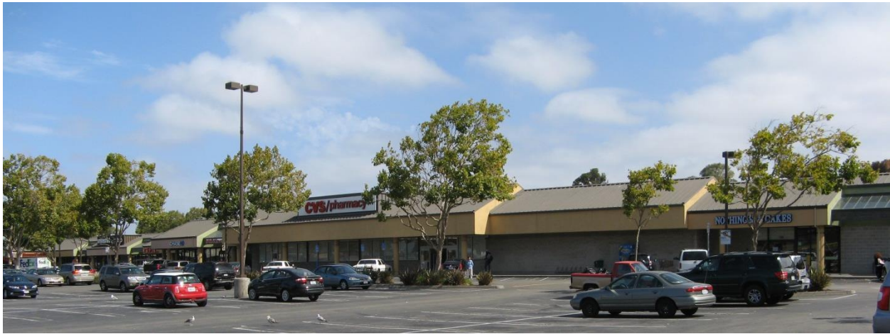
CVS Pharmacy, owned by Weingarten Realty but not included in the proposed project.
