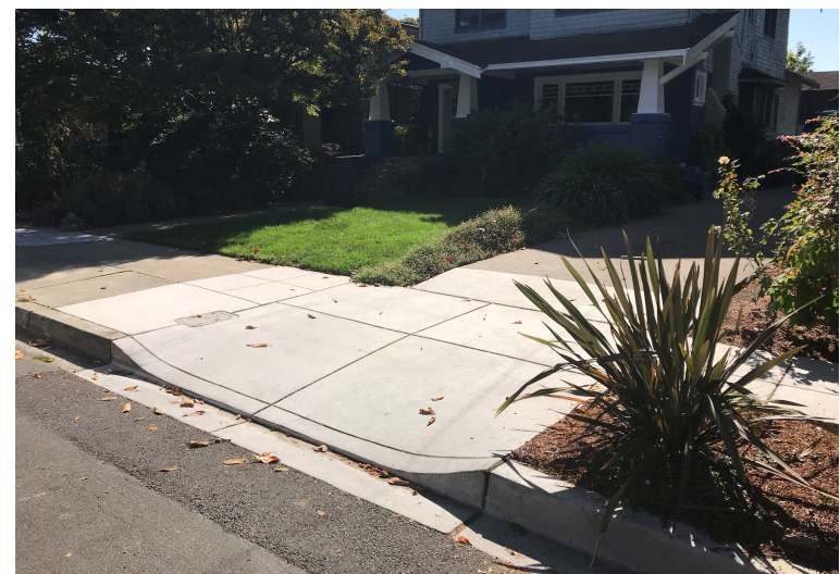
Driveway / Sidewalk Repair
