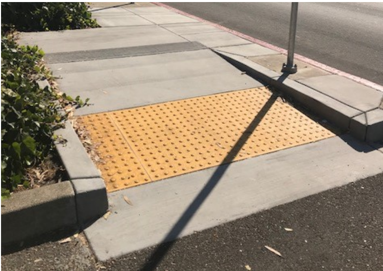
Curb Ramp Construction
