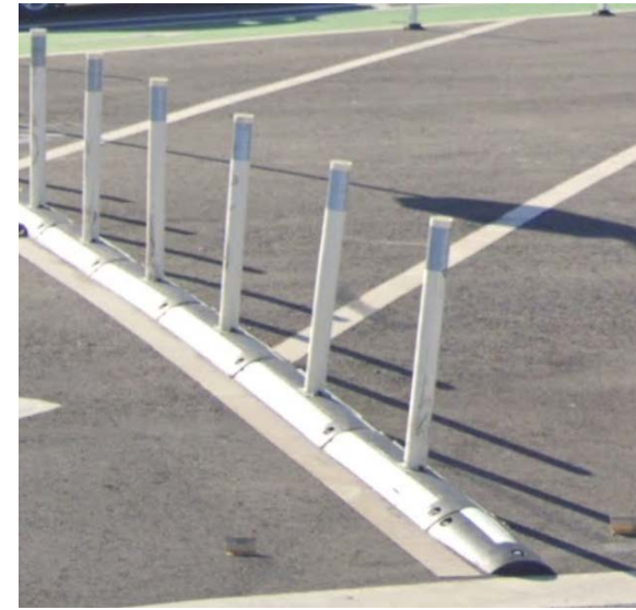
Delineators on duracurb: ~$100/LF
