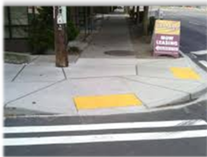
Accessible Curb Ramps
