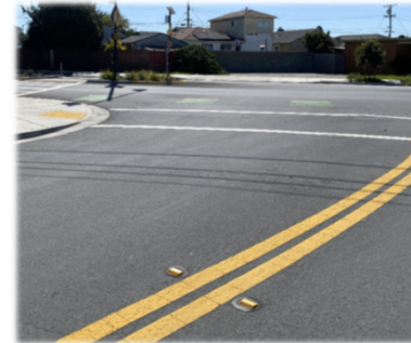
Pavement Surface Seal
