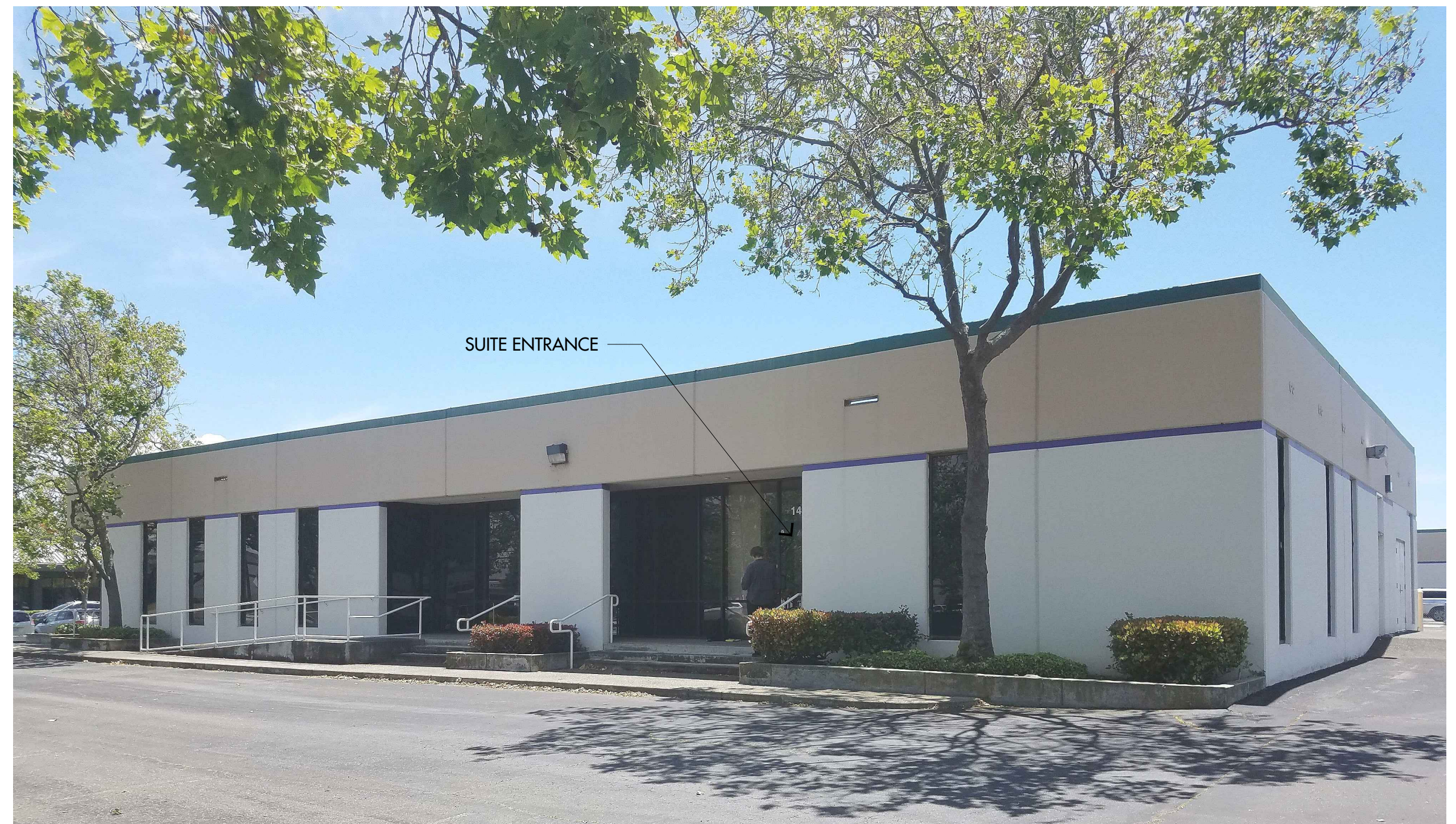
4 PHOTOGRAPH LOOKING SOUTH AT SUITE ENTRANCE NO SCALE
