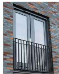
① JULIET BALCONY WITH METAL RAILING
