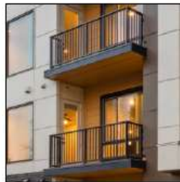
① VERTICAL RIBBED METAL RAILING
