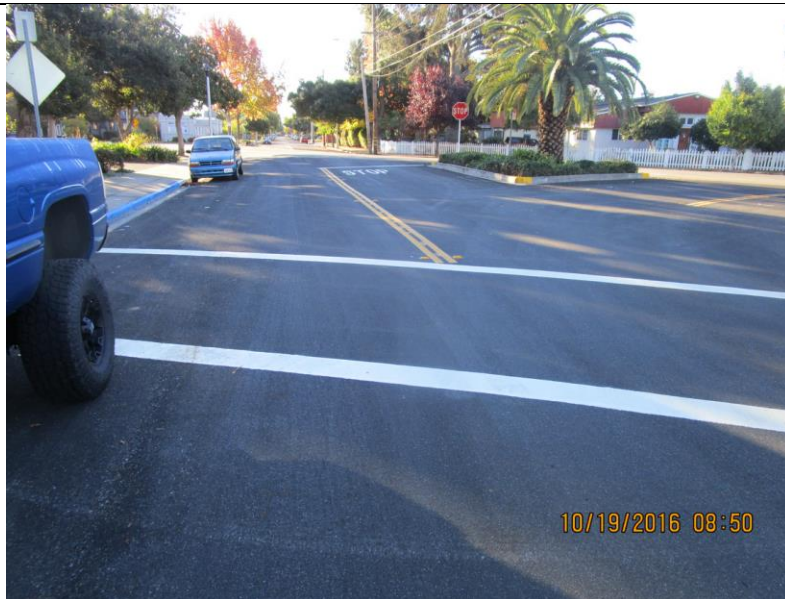
COMPLETED SLURRY SEAL ON BREED AVENUE
