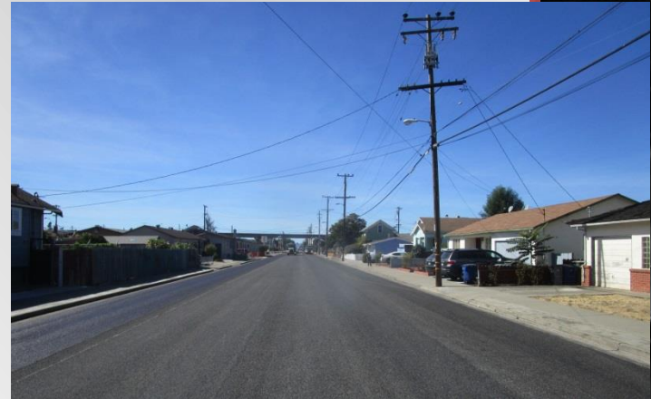
Williams St Slurry Seal
