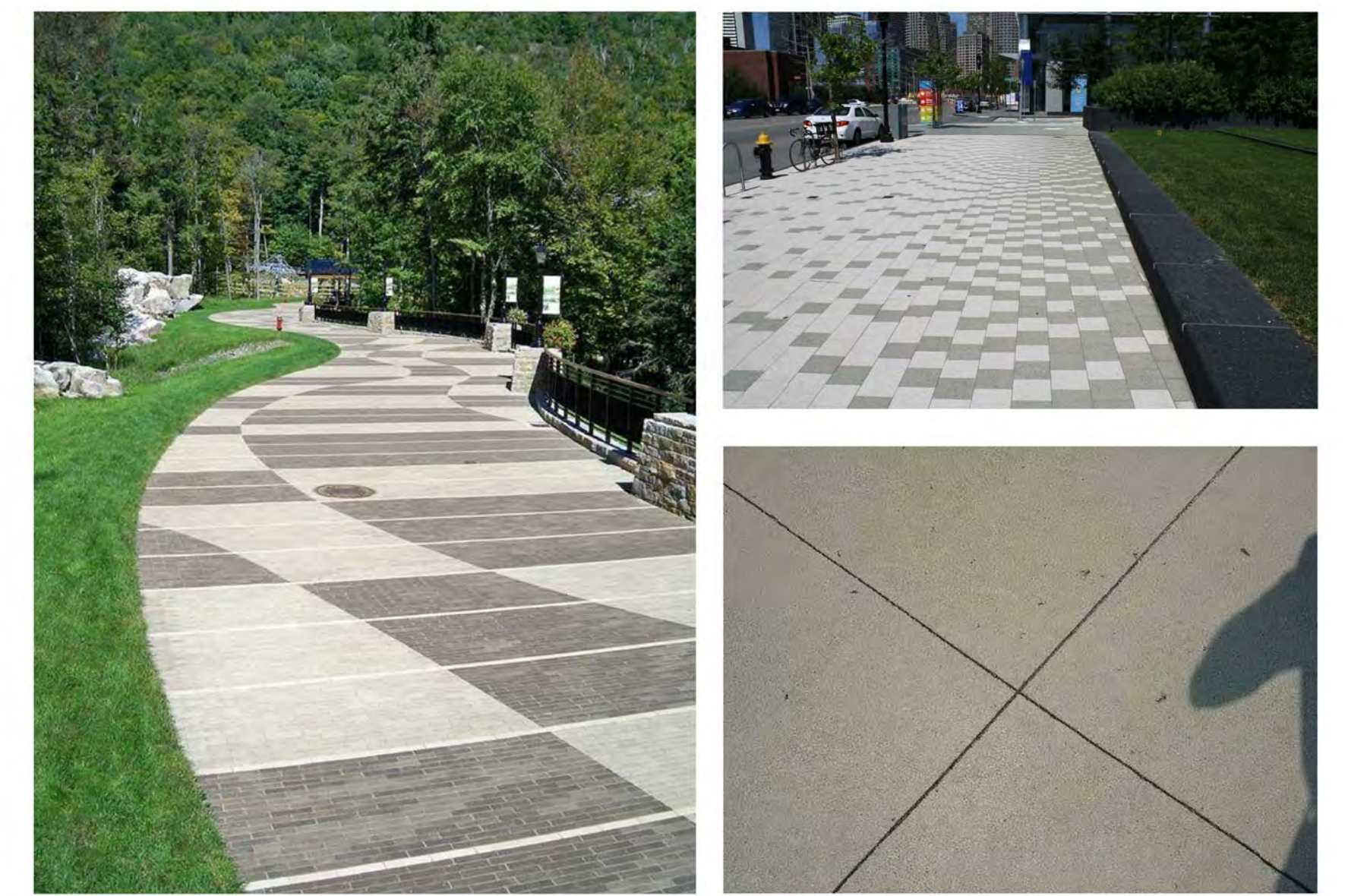
ENTRY PLAZA PAVING: TWO TONES OF COLORED CONCRETE
