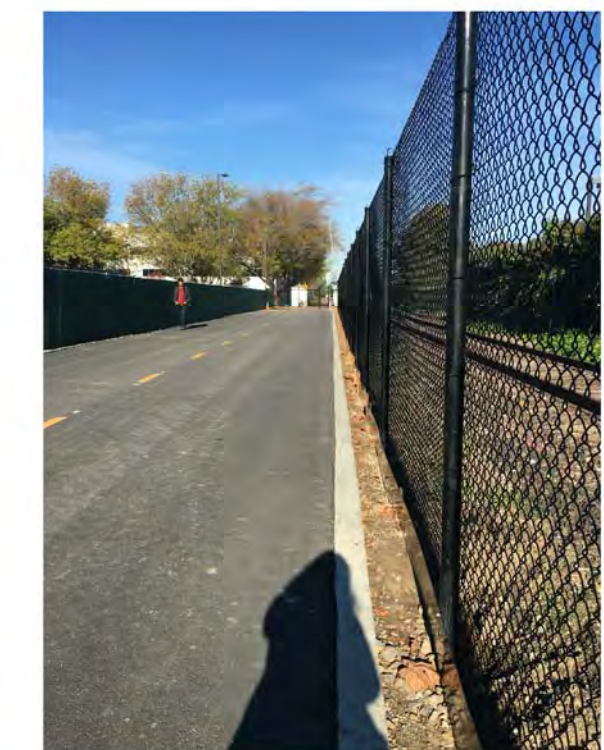
FENCE AT PERIMETER: UPRR AND SPRR EDGES, 8" TALL VINYL CLAD CHAIN LINK
