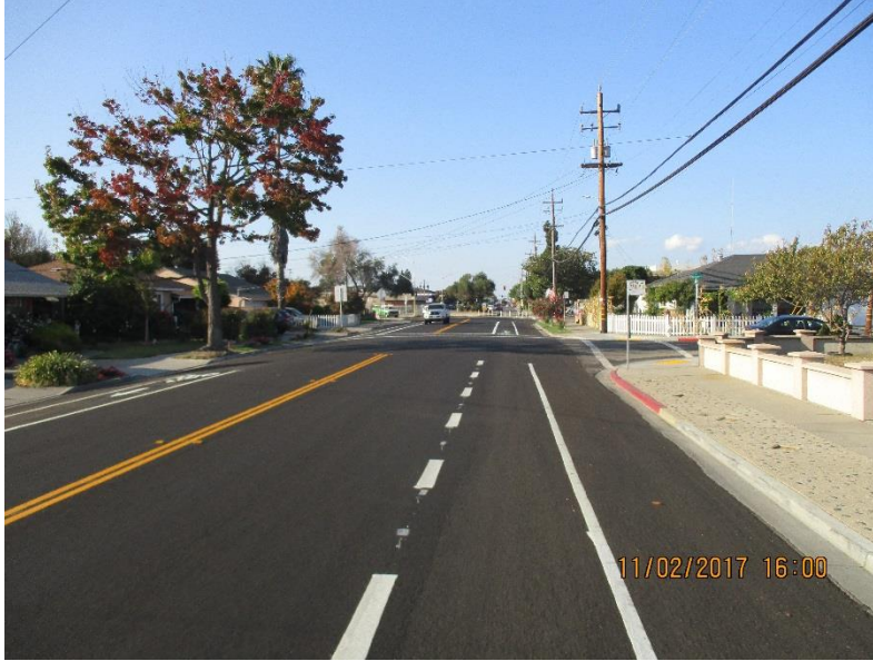
COMPLETED CAPE SEAL WITH NEW BIKE LANES ON MERCED STREET
