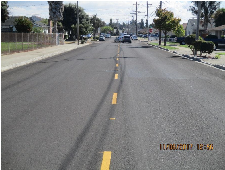
COMPLETED SLURRY SEAL ON MONTEREY BOULEVARD
