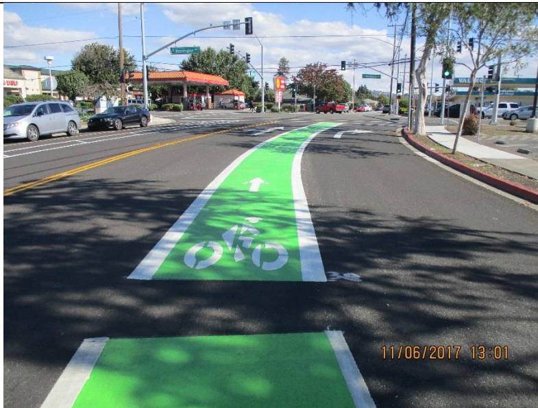
COMPLETED MICRO SEAL WITH NEW BIKE LANES ON MONTEREY BOULEVARD
