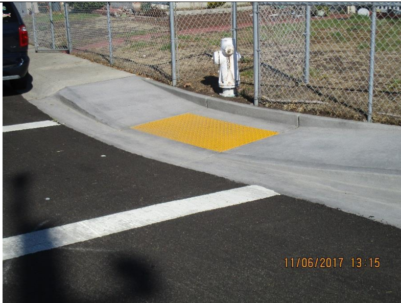
UPGRADED CURB RAMP AT PURDUE-ESSER
