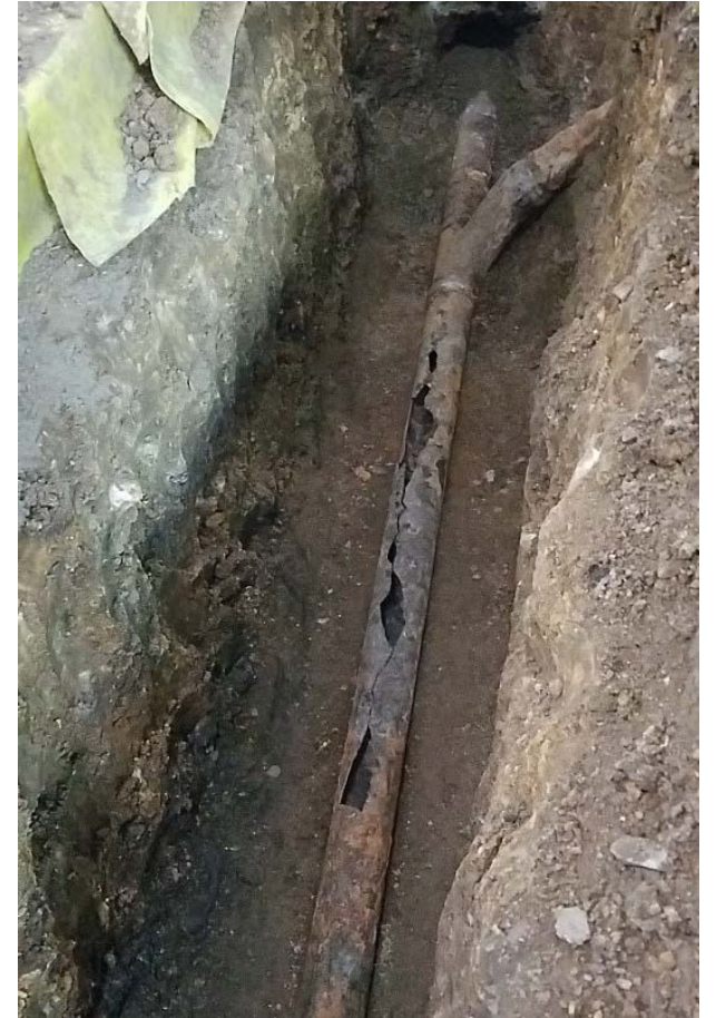
Unforeseen pipe deterioration at B&G Club Pool
